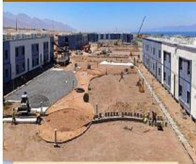
5K PROJECT HAQL NEOM COMPOUND NESMA & PARTNERS
